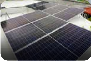
INSTALLATION OF SOLAR PANELS
